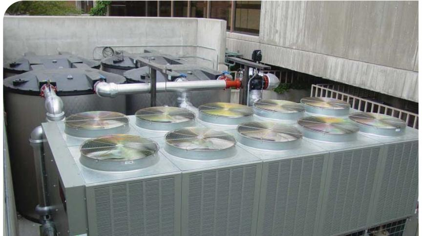
Trane reduces energy costs by incorporating an ice storage system design that uses ice made at night, when energy demand and cost are lowest, to cool the building during the day.
